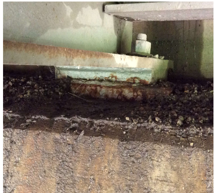
PHOTO 2 Description Bent 1. Beam 5. Bearing corrosion.
