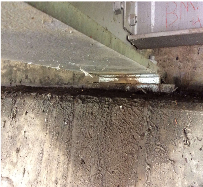
PHOTO 1 Description Bent 4. Beam 3 bearing is fretting.
