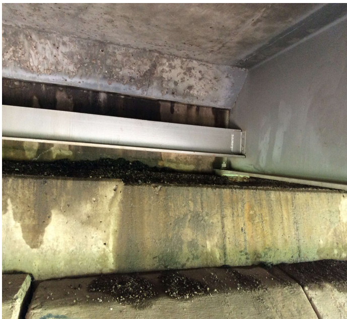
PHOTO 3 Description Bent 1 debris on cap.
